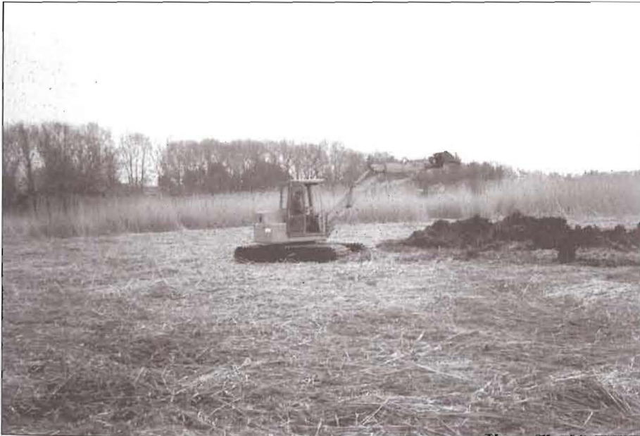
Fig. 10 A low-ground pressure excavator digging a creek during the restoration of a buried marsh. (R. Rozsa)
