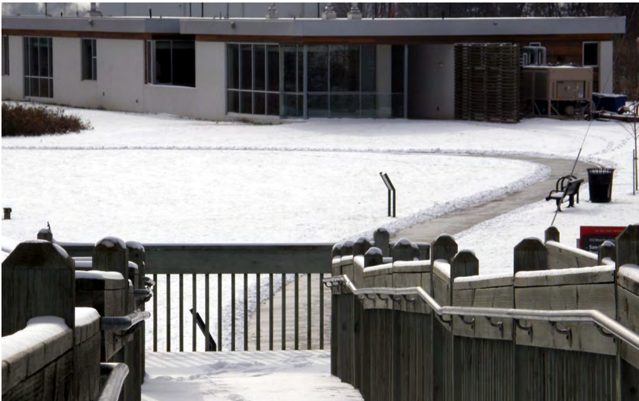
Snow outlines the Sandefur Wetland Pavilion and the Heffner Wetland Building in a winter scene.
