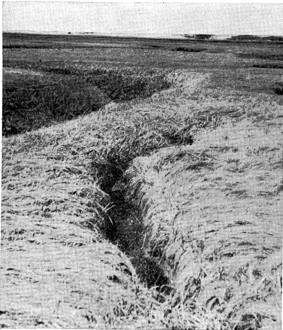
FIG. 46. A crack in the marsh surface due to the slumping of the bank of Navigation Creek. Spring 1955. The crack is about 1 ft wide and 30-40 ft long.
