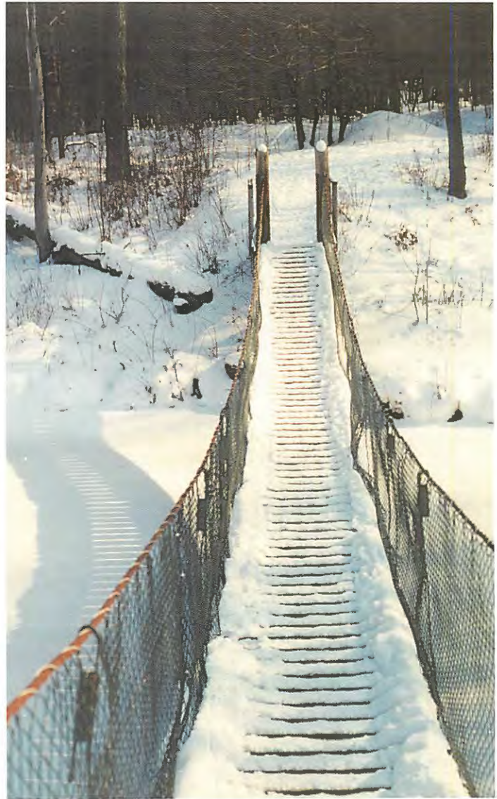
Swinging bridge over the West Branch. Photo by Patricia Spicer.
