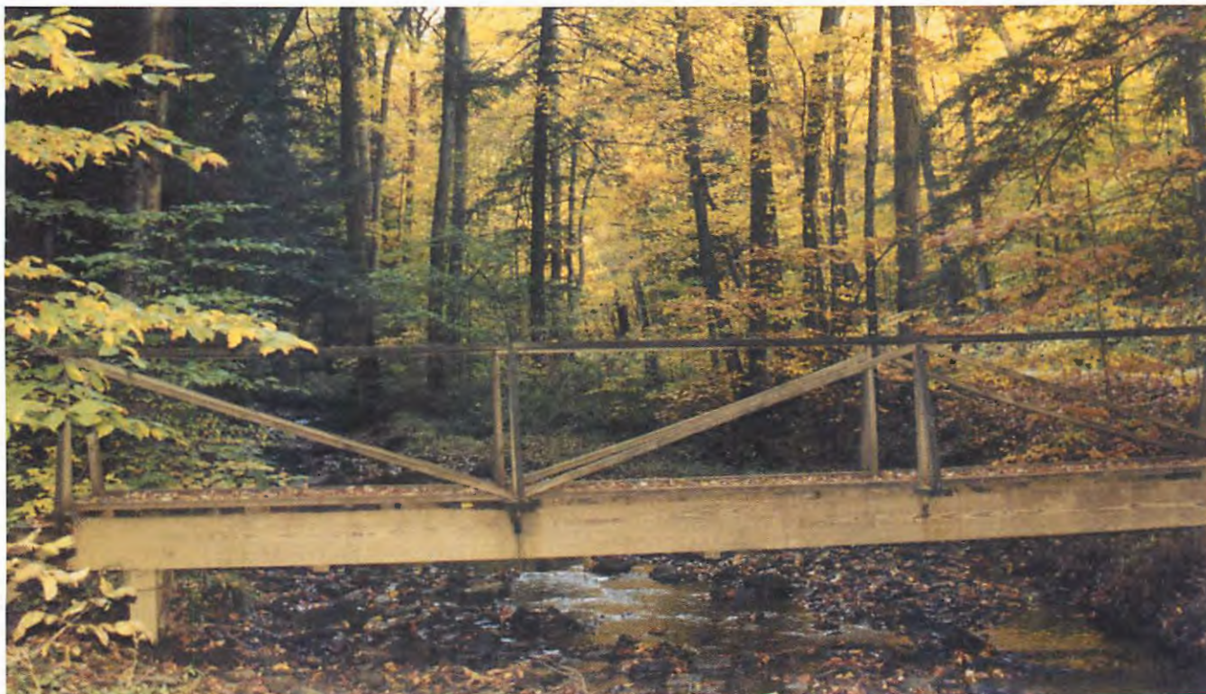
Footbridge over Anders Run. Photo by Ryan Butryn.
