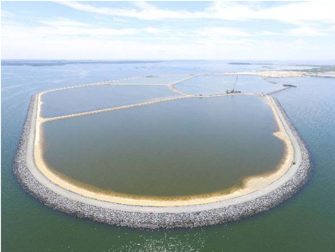
Drone Imagery of the Poplar Island Expansion wetland cells and open water embayment.
