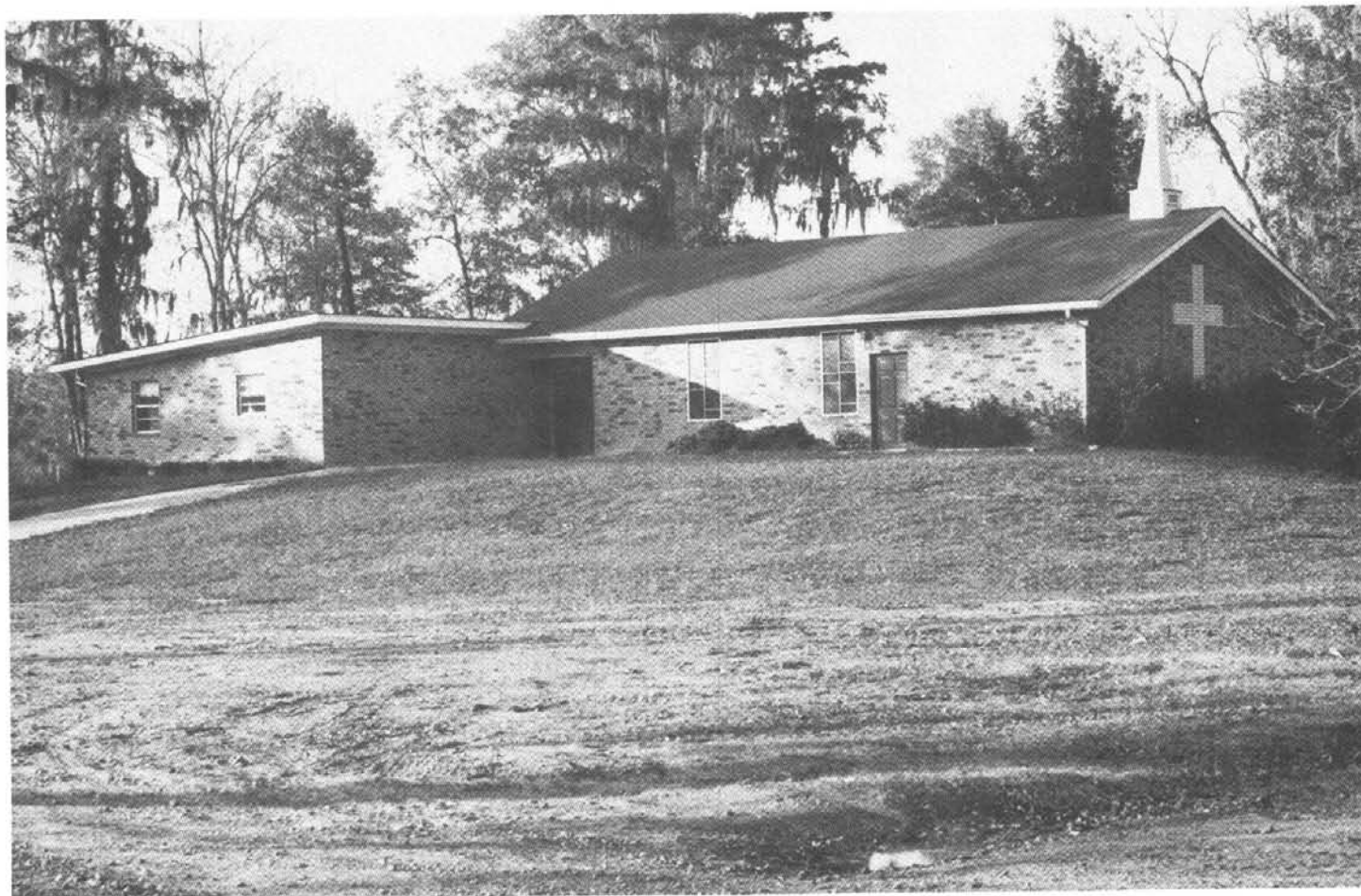
Figure 2.—This building in an area of Dundee silt loam, 0 to 1 percent slopes, is on a properly constructed mound of soil material that is above the expected flood elevation.
