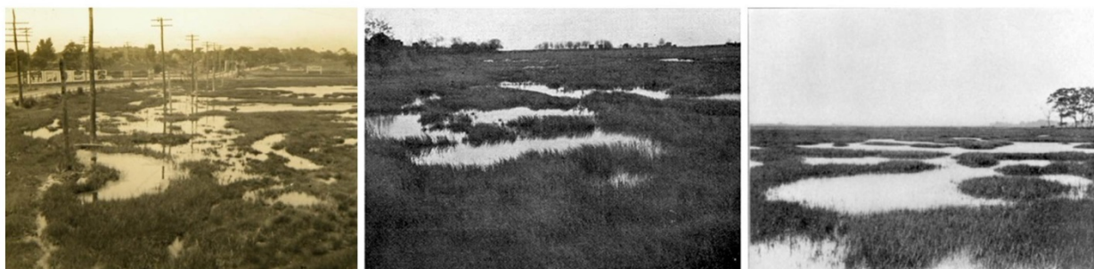
Figure 15. Historic photographs showing the abundance of open water panne habitat in three tidal marshes in Connecticut prior to ditching. From left to right: Quinnipiac River marsh (1917), marsh near Morris Cove (~1915) and Westbrook (Nichols, 1920). The first two images are from DEEP archives.
