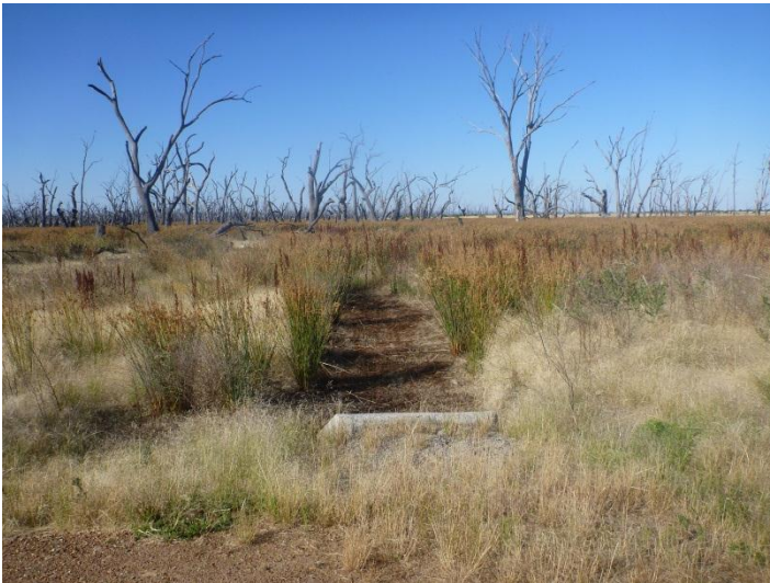
Fig. 3-8 The western side of the culvert draining under Ashmeads Road towards the western side of the wetland.
