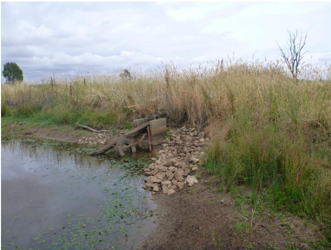
Fig. 3-2 The outlet pipe and levee at 7 Mile Wetland.
