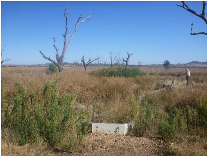
Fig. 3-72 The culvert under the Winton North Road looking west.
