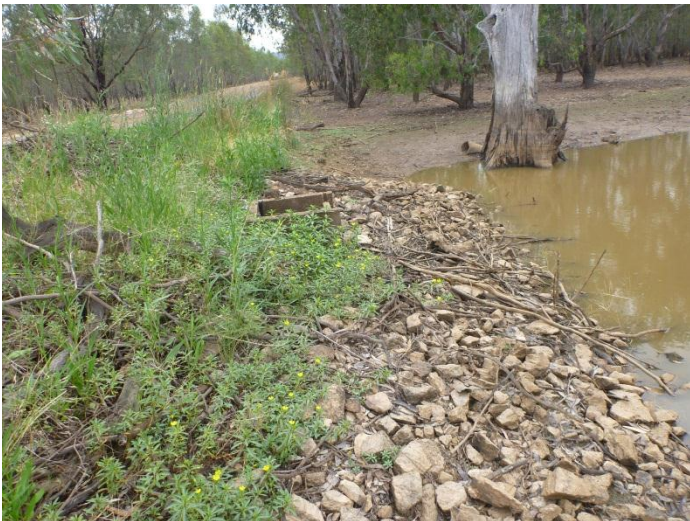
Fig. 3-5 The outlet pipe and track embankment at 11 Mile Wetland.
