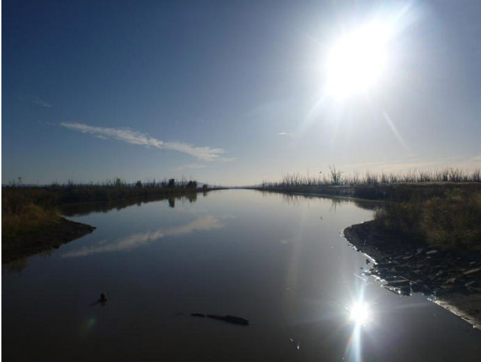
Fig. 3-42 The outlet channel from Sergeants Swamp from the dam wall looking east.
