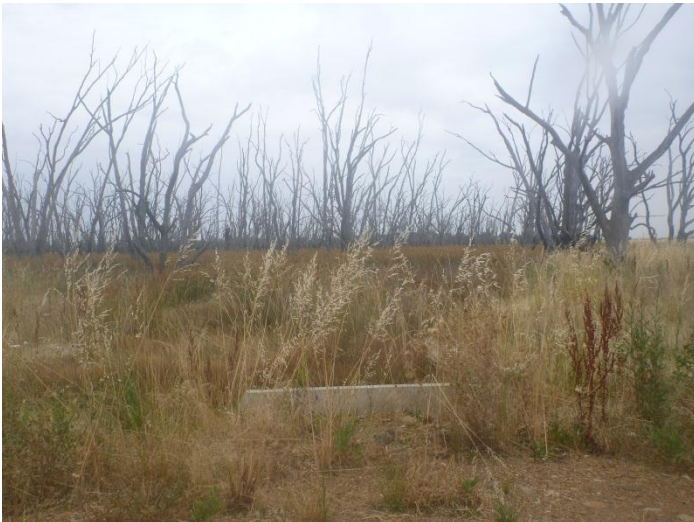
Fig. 3-31 The outlet culvert under 11 Mile Track looking towards Humphries Swamp.
